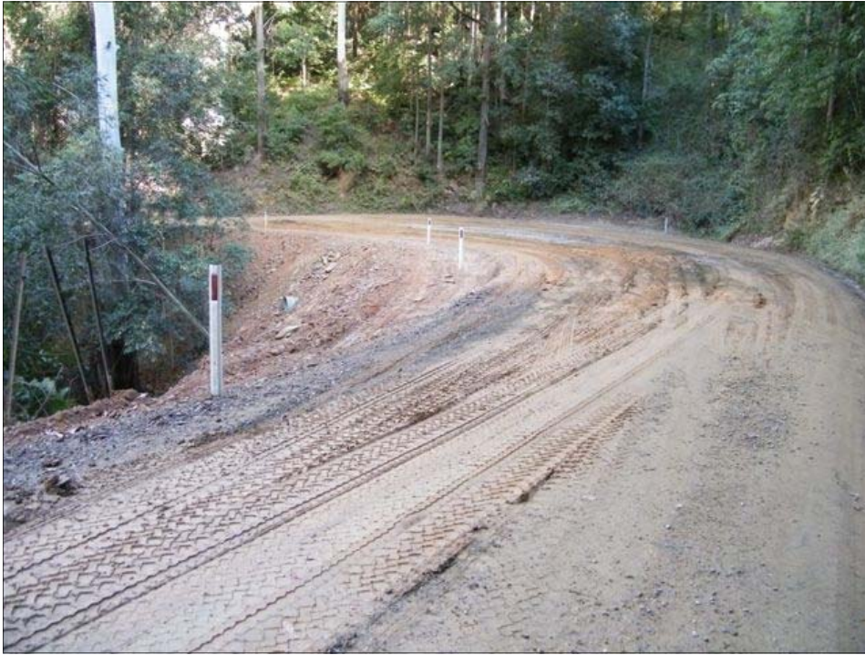
TAYLORS ARM ROAD AT 51.2KM—LANDSLIP RESTORATION
