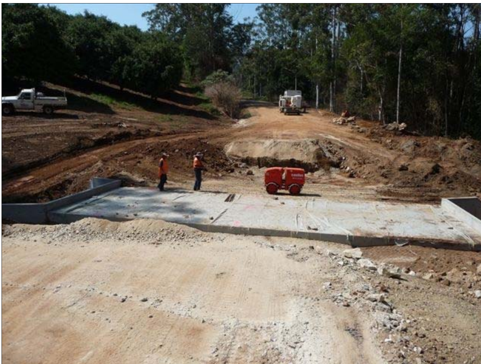
EAST-WEST ROAD—REPLACEMENT OF CULVERT
