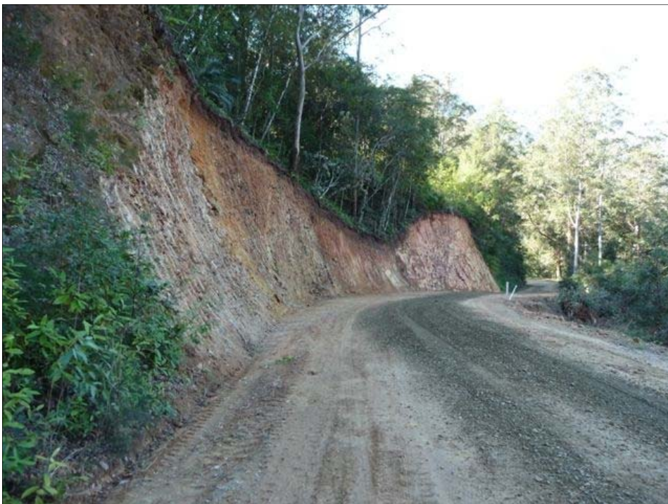
TAYLORS ARM ROAD AT 53.6KM—LANDSLIP RESTORATION
