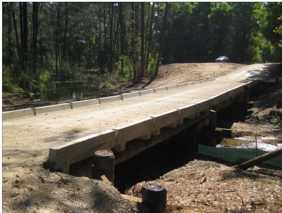
MORANS ROAD—REPLACEMENT OF BRIDGE
