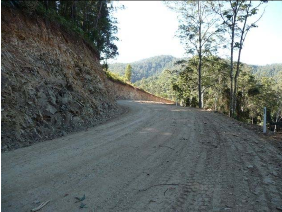
TAYLORS ARM ROAD AT 48.7KM—LANDSLIP RESTORATION
