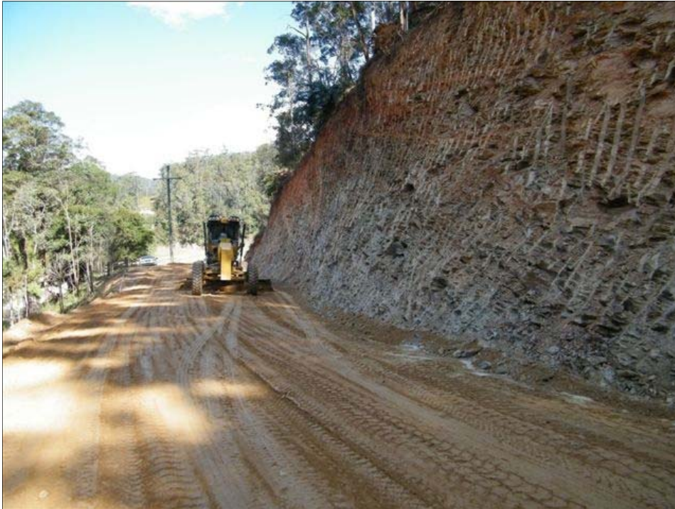
TAYLORS ARM ROAD AT 54.4KM—LANDSLIP RESTORATION
