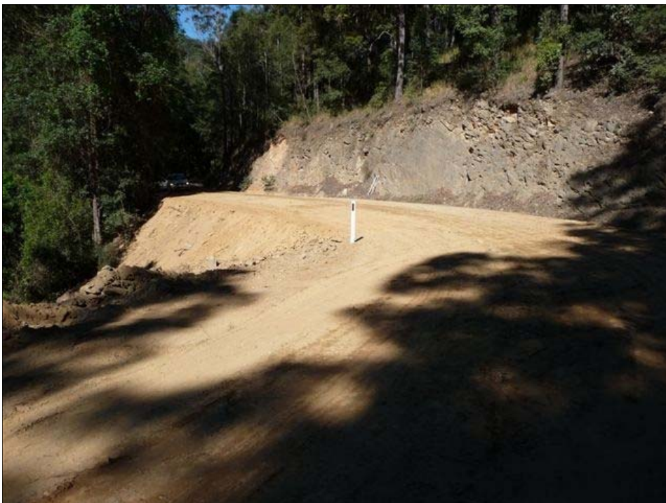
TAYLORS ARM ROAD AT 50.9KM—LANDSLIP RESTORATION
