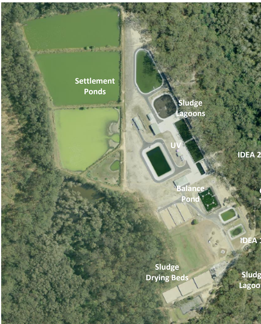
Figure 9-5: Aerial view of Nambucca Heads STP
