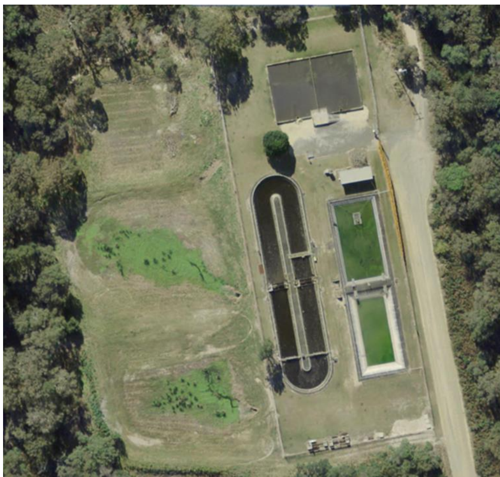
Figure 8-5: Aerial view of Scotts Head STP
