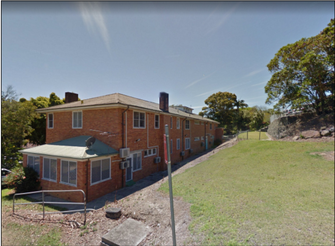
Figure 8: Current view of accommodation quarters from Nancye Roberts Drive.
