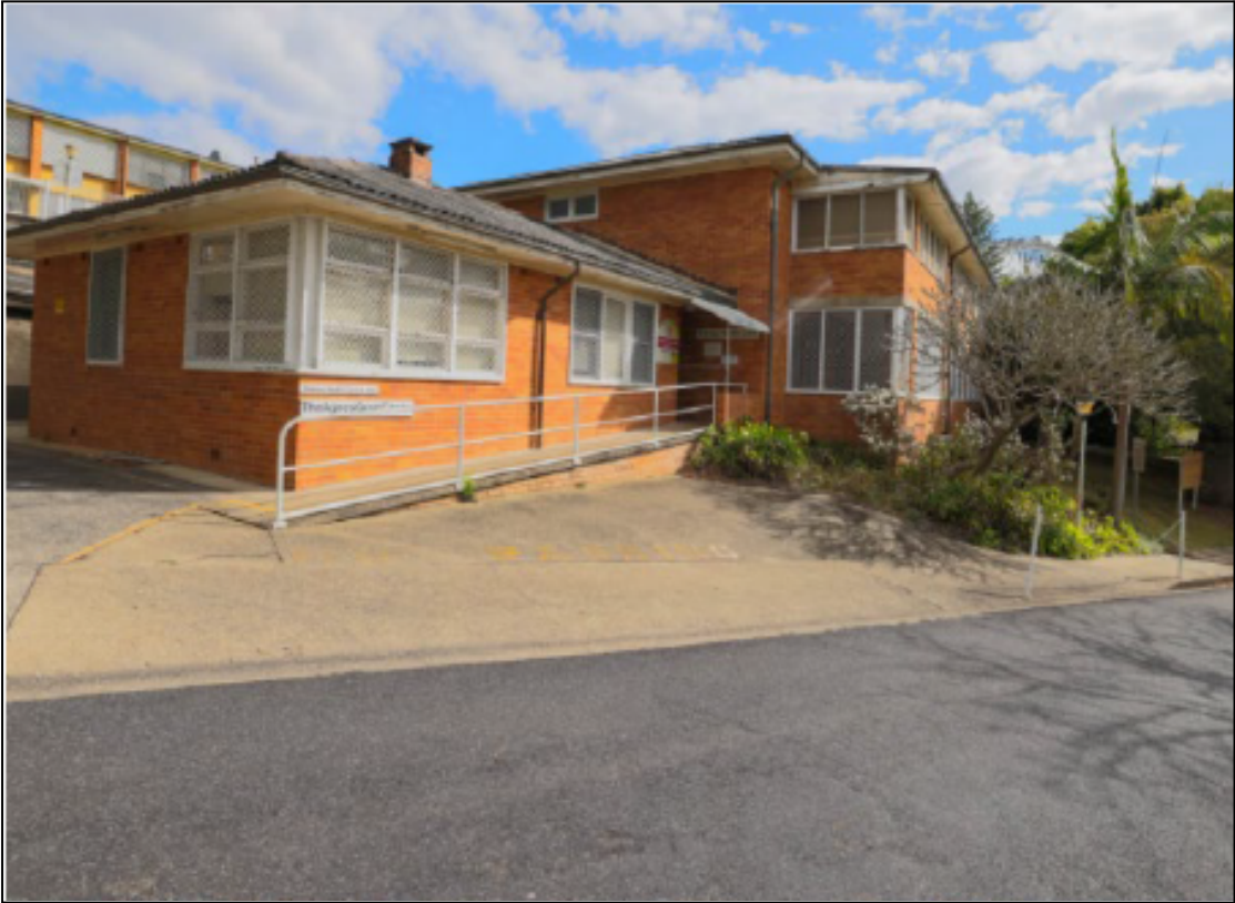
Figure 12: Current view of administration/accommodation building fronting Boundary Street.
