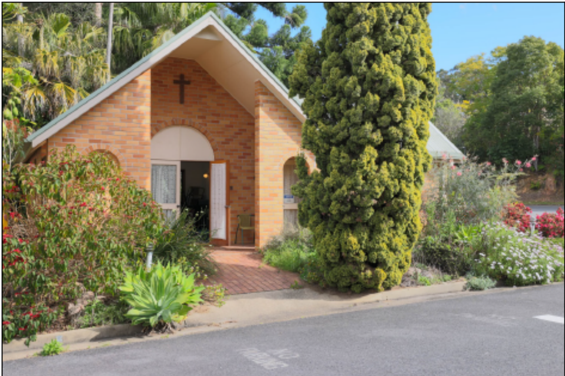
Figure 15: View of the current chapel.
