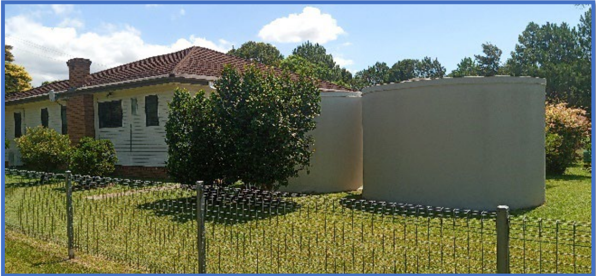
Figure 12: 2 x ~20,000 L. concrete tanks
