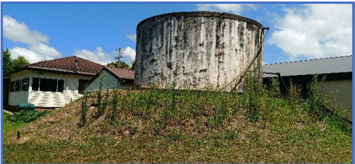
Figure 13: 1 x ~20,000 L. concrete tank
