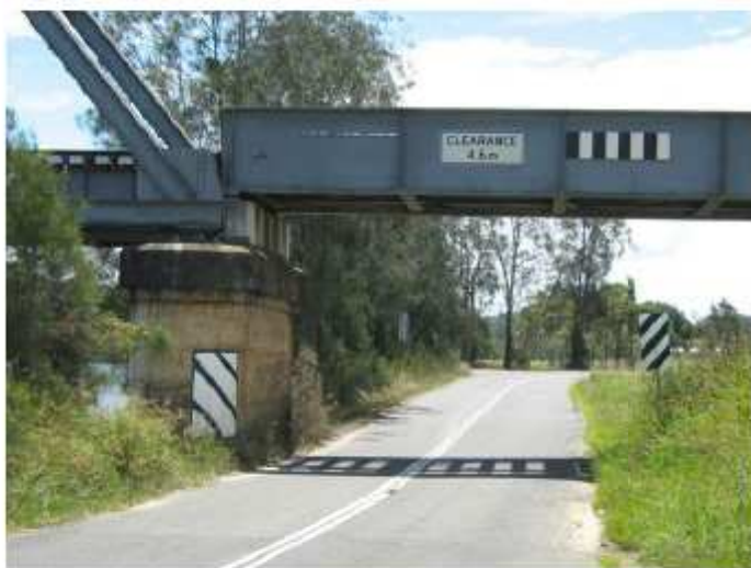
Figure 5 First rail underpass with deficient signage.
