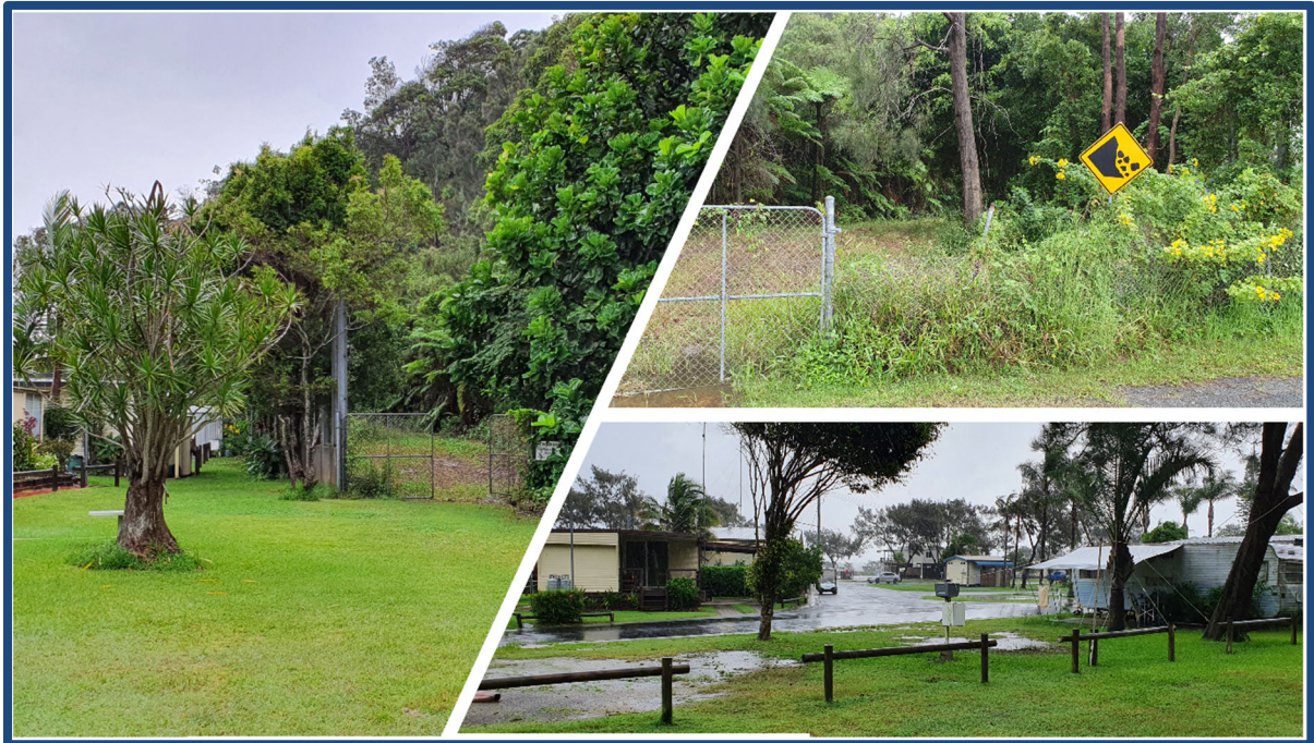
Figure 20 – Wellington Park Assets – Fencing Steel and wire fencing at quarry exclusion (left); Treated pine boundary fence between White Albatross Holiday Park (bottom right).
