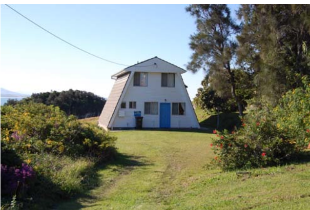
Example of varied building form
