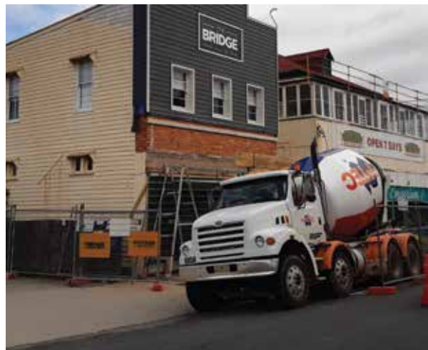
Actual verandah post re-instatement works underway
