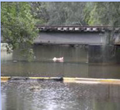
Flooding in Cow Creek February 09 Photo NSC
