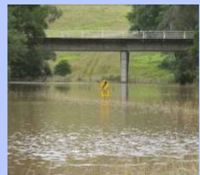
Flooding on Scotts Head Rd April 09 Photo NSC
