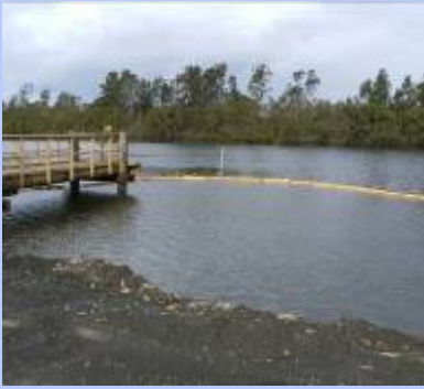
Sediment Skirt Used to Protect Aquatic Environment Photo NSC
