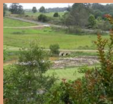
Dam Building Photo NSC
