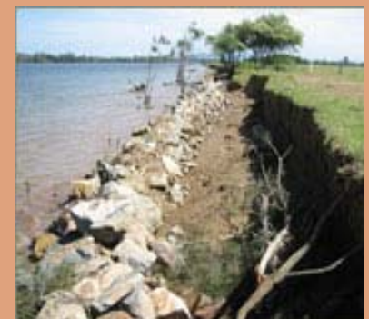
Rock Fillet Bank Restoration Work Photo Landcare
