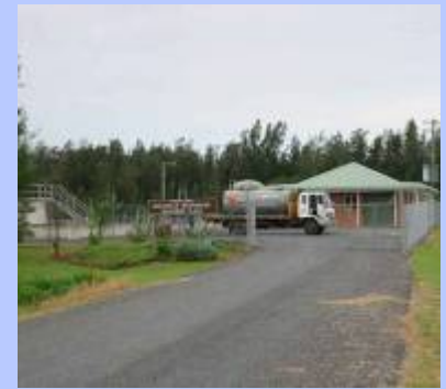
Macksville Sewage Treatment Plant Photo NSC
