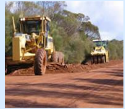
Clearing Vegetation for a fire break Photo Google
