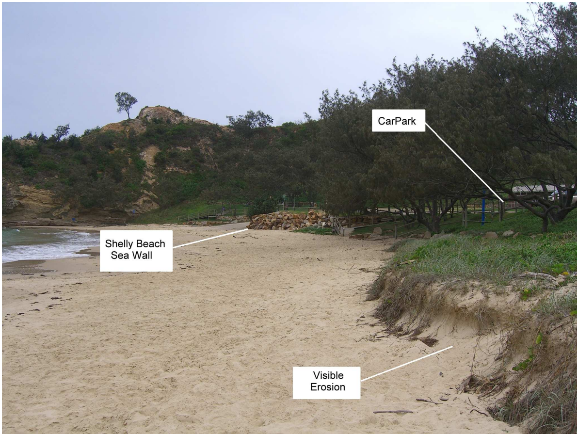
Figure A.11 - Shelly Beach (Block 3) looking South
