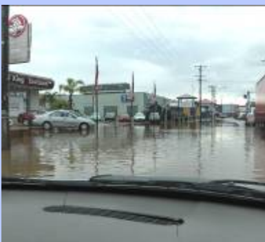
Flooding in Cooper St - Macksville Photo NSC
