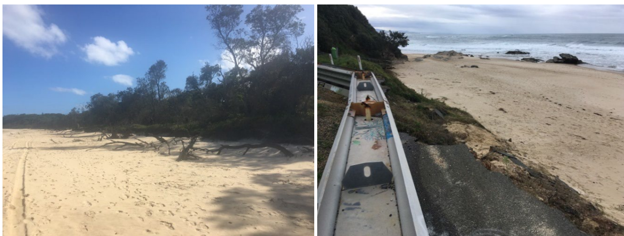
Plate 8: Left: Vegetation debris on receding shoreline north of Swimming Creek entrance (December 2018); Right: recession of beach at Ulrick Drive carpark (north end of Beilby's Beach) causing undercutting and collapse of the road surface (July 2018)
