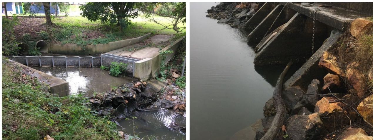
Figure 7: Left: Gross Pollutant Trap at Bellwood Park; Right: damaged floodgate at East Street, Macksville (July 2018)
