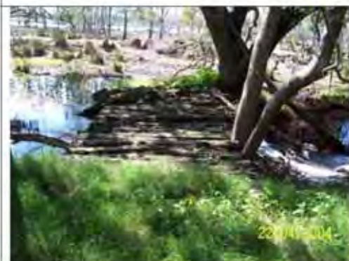
Old farm crossing acts as weir (0.5 m high) - limits tidal inflows and retains upstream water levels ( Dyer ) ( Mangroves )
