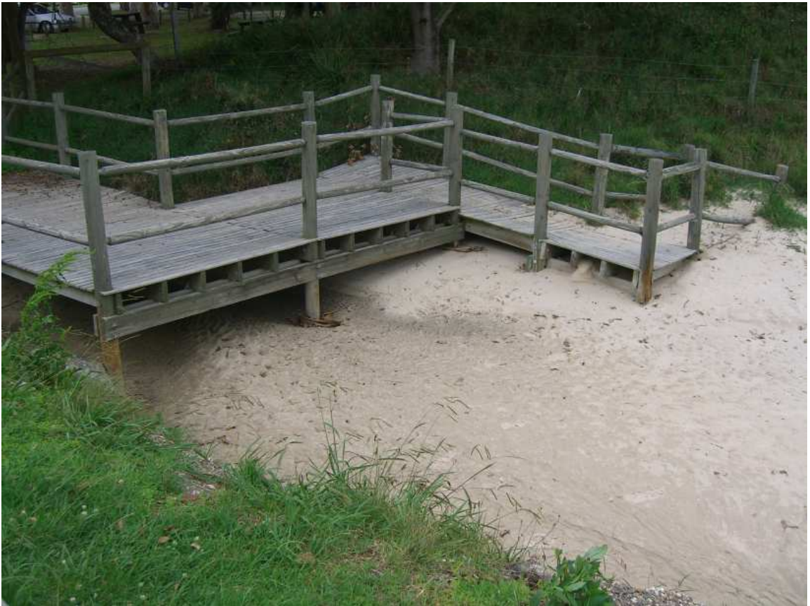
Figure 3.2 – Stormwater drain adjacent to carpark, southern end Forster Beach
