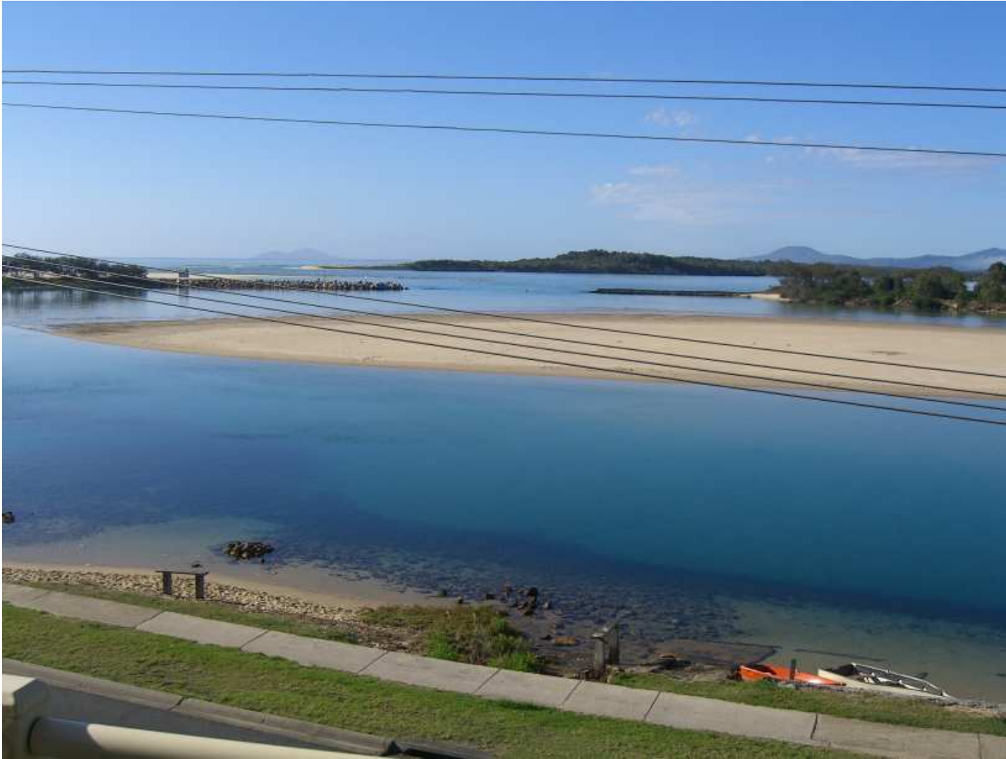
Figure 3.7 – Gap in the northern breakwall, Nambucca Heads
