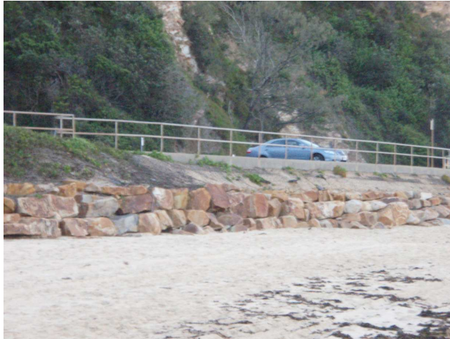
Carpark seawall, Main Beach October 2008
