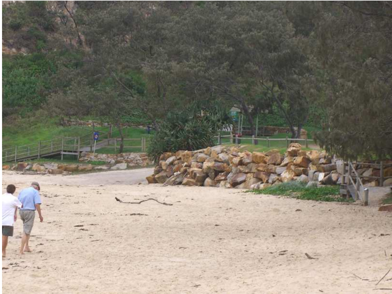
Figure 3.10 – Seawall and boat ramp, Shelly Beach
