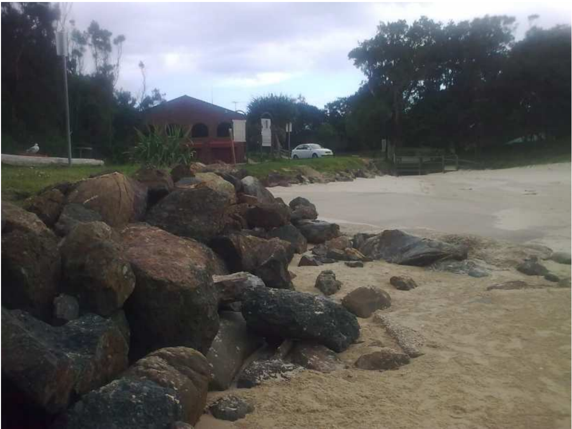
Figure 3.4 – Seawall adjacent to surf club, Forster Beach
