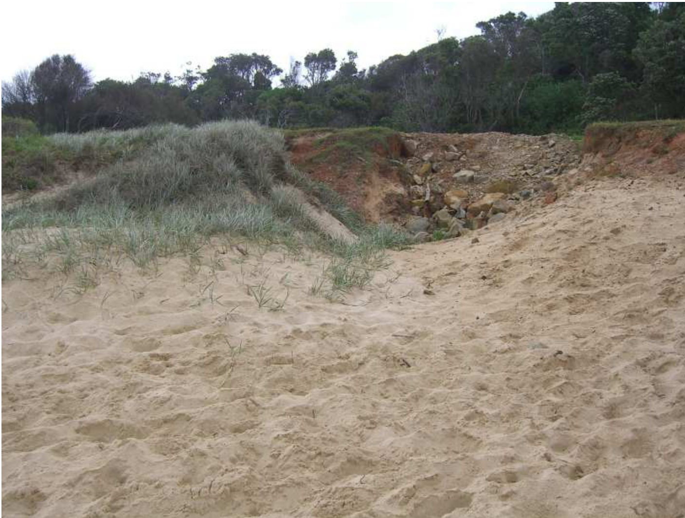
Figure 3.11 – Erosion at Beilbys Beach carpark
