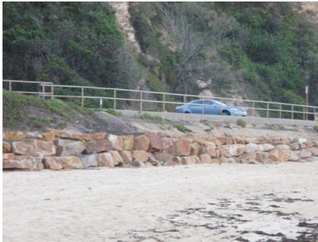
Carpark seawall, Main Beach October 2008
