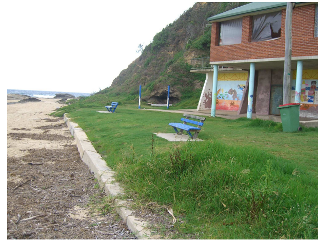
Main Beach surf club with concrete retaining wall in foreground
