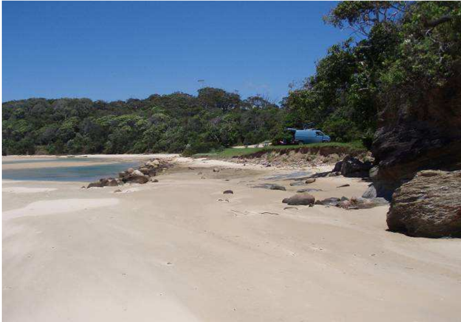
Figure 3.14 – Erosion at South Valla Beach carpark caused by creek entrance dynamics, December 2008
