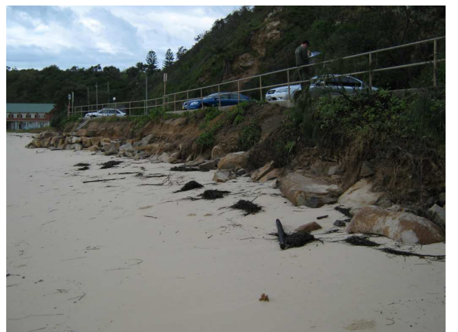
Carpark seawall, Main Beach May 28 2009
