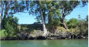
The highway/river interface at this location is extremely narrow with a steep river bank profile. There is undermining of the river bank edge and informal access down the bank is adding to erosion. The western side of the highway is more suited to pedestrian access and has the potential for new tree planting. Large trees along this section of steep bank add to the bank stability and the visual amenity of this foreshore location.
