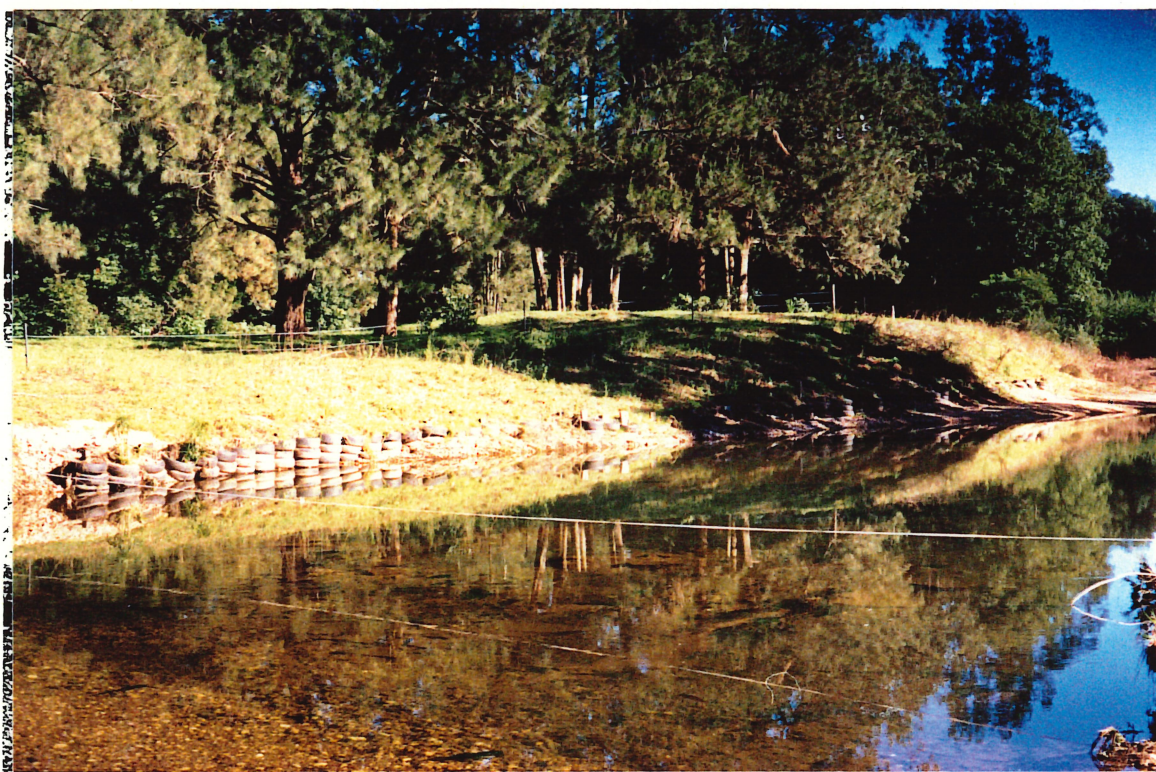
Plate 3.17: Tyre wall on Missabotti Creek (M3). The wall survived the floods of May 1996.
