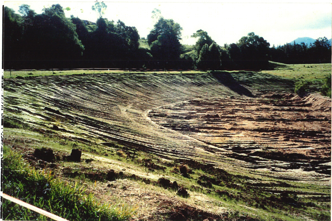
Plate 3.16: Upstream view of an eroded bank on Missabotti Creek (M4). (a) (above) Prior to realignment works in November 1996. (b) (below) after realignment work in April 1997.
