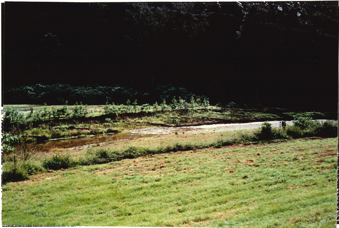
Plate 3.8: Brush groynes on upper North Arm (upstream of N2) in June 1997. These groynes have survived a number of floods since construction in late 1995.
