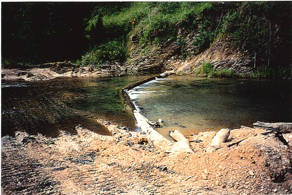
Plate 3.3: Log sill constructed at Argent's Hill (N3). April 1996.
