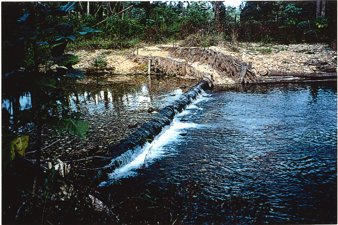
Plate 3.1: Straight log sill on Taylors Arm (downstream of T3). June 1997.
