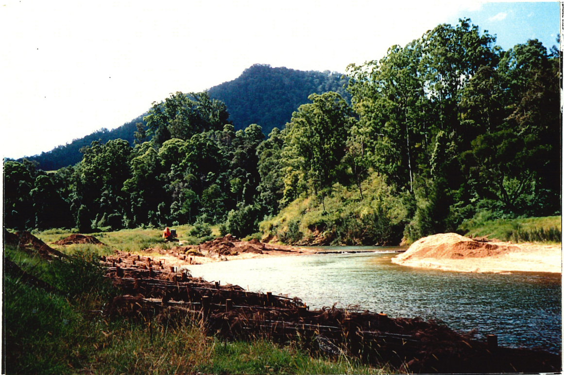
Plate 3.7: Brush groynes constructed at Argent's Hill (N3) on North Arm. (a) (above) just after construction in April 1996. (b) (below) after the flood of May 1996.
