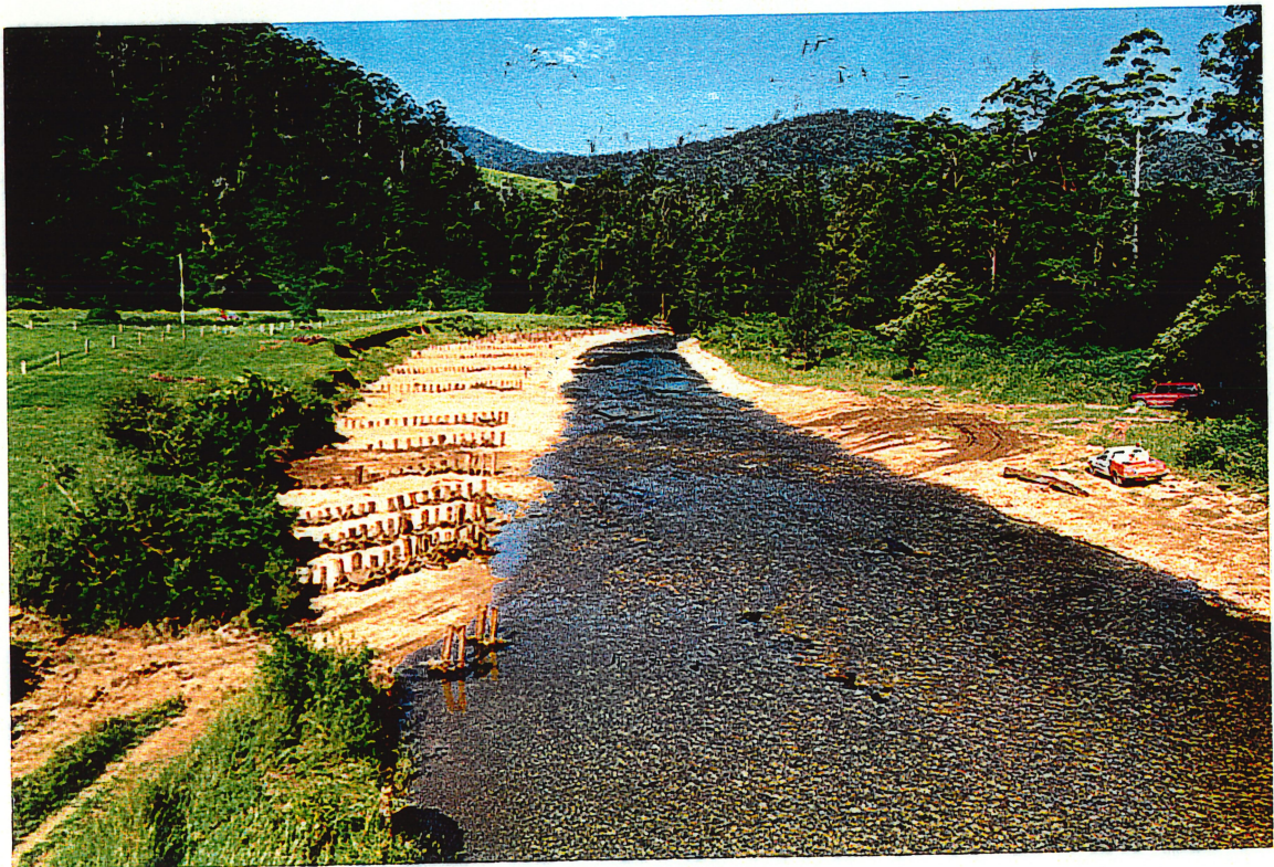
Plate 3.9: Pin groynes on Taylors Arm (between T2 and T3). (a) (above) Eroding bank in February 1996. (b) (below) after pin groyne construction in February 1997.
