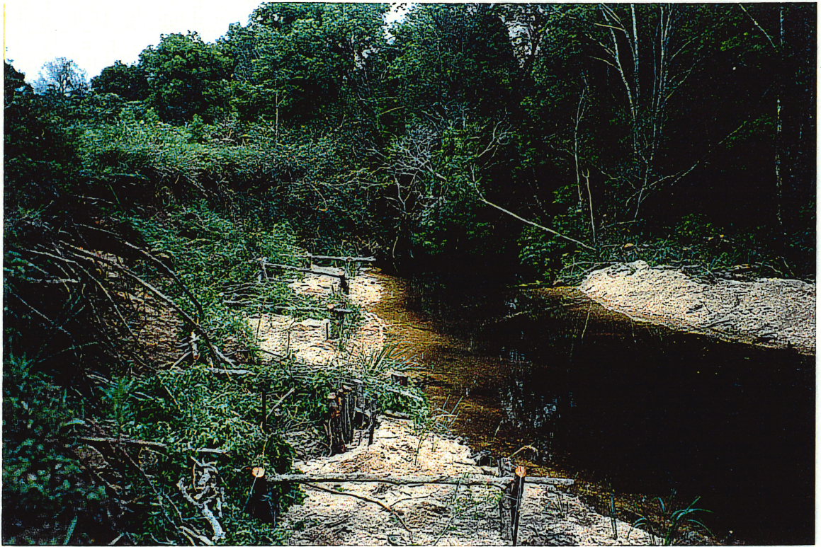
Plate 3.10: Jacks constructed by the Jobskills team at Deep Creek near Valla (upstream of D3). February 1997.
