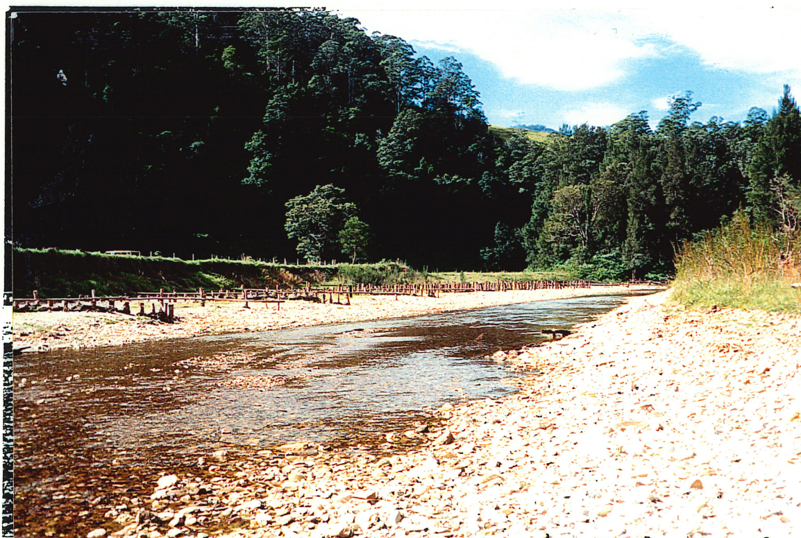
Plate 3.6: Downstream view of an eroded bank on Taylors Arm (between T2 and T3). (a) (above) In February 1996 before groynes were built, and (b) (below) June 1997 after the groynes were completed.
