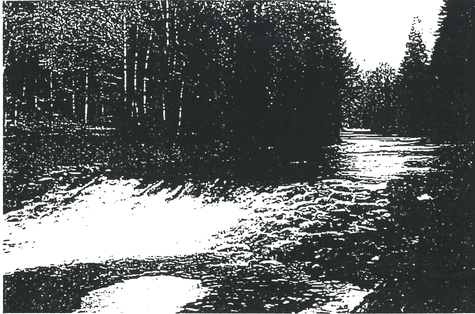
Plate 3.12: An example of the rock ramps used in Bavaria, Germany to control bed levels.
