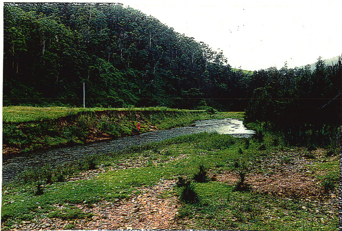
Plate 3.6: Downstream view of an eroded bank on Taylors Arm (between T2 and T3). (a) (above) In February 1996 before groynes were built, and (b) (below) June 1997 after the groynes were completed.
