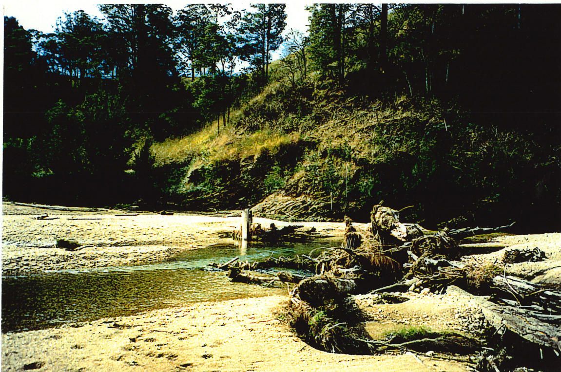
Plate 3.4: Log sill at Argent's Hill (N3) after the May 1996 flood. Undercut and outflanked
